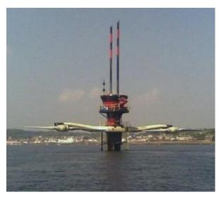
Figure 4 - MCT's Seagen Tidal Turbine in Strangford Lough<sup>22</sup>.
